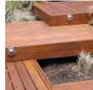
Timber decks and walkways
