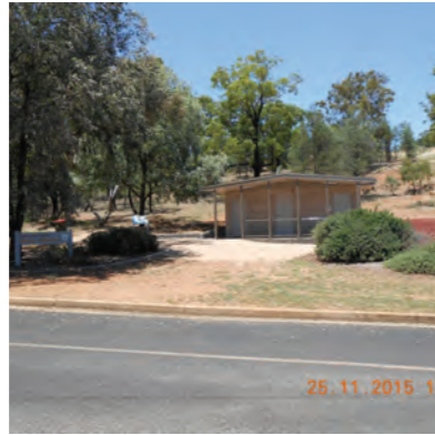
View toward existing amenity block
