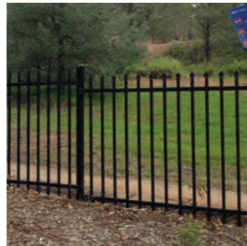
Amenities and changing room structure
