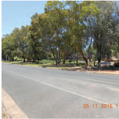
Bushman Rd approach to project site.
