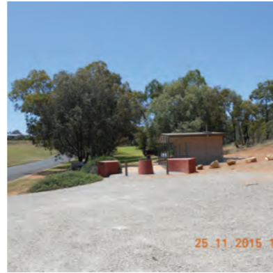
View from existing car park toward entry into park
