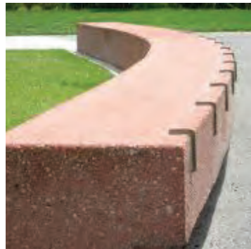
Formed concrete seating walls
