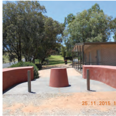
Existing entry feature/gateway
