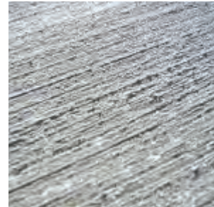
Concrete: Broom finish
