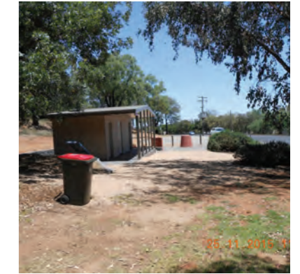
View towards the existing amenities block
