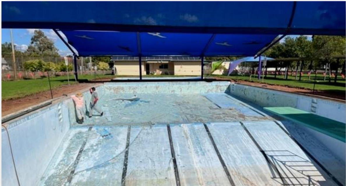
Photo 16 Trundle Pool refurbishment works in progress.
