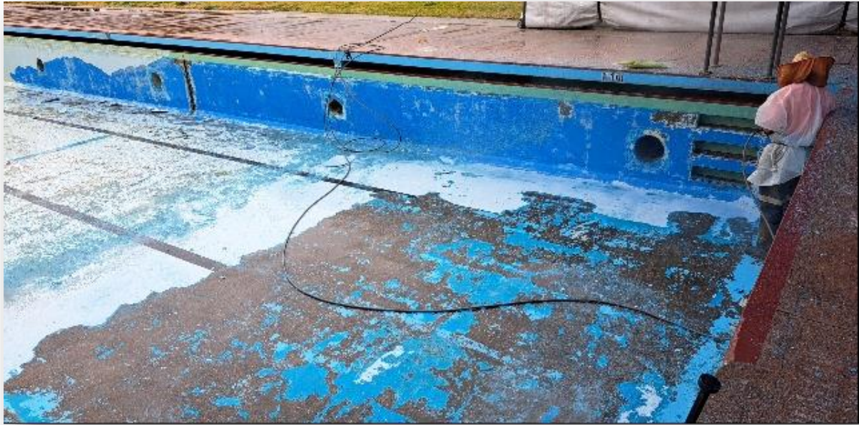
Photo 24 Sand blasting of the Peak Hill pool shell.
