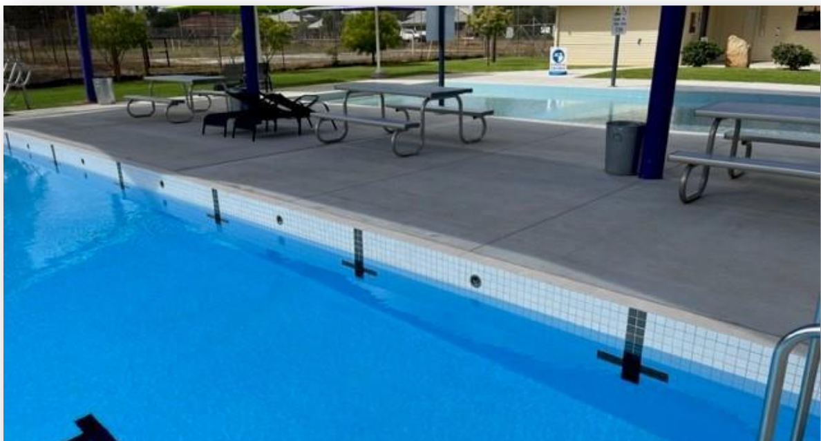
Photo 17 Trundle Pool refurbishment works complete.
