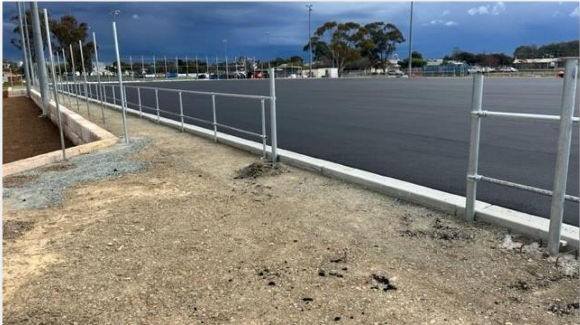
Photo 10 Reconstruction of Stephen Davies Field - bitumen base.
