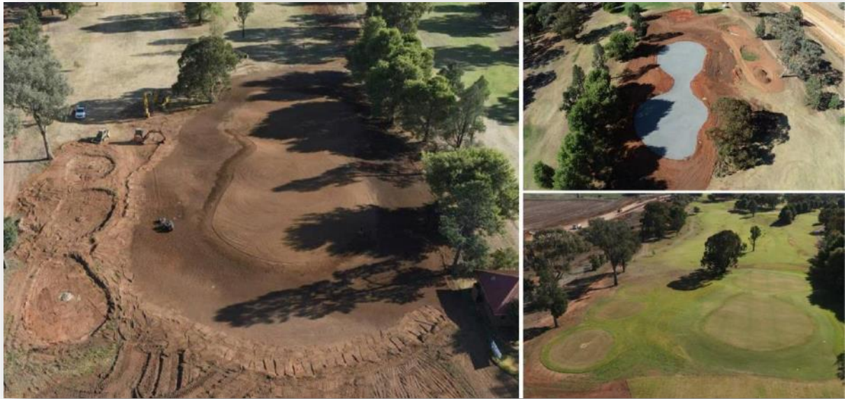
Photo 19 Re-construction work at the Parkes Golf Course (Champion Post).
