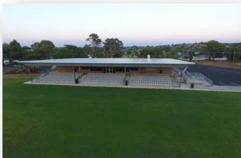
Photo 9 Spicer Oval Grandstand and Amenities (Heinz Constructions)
