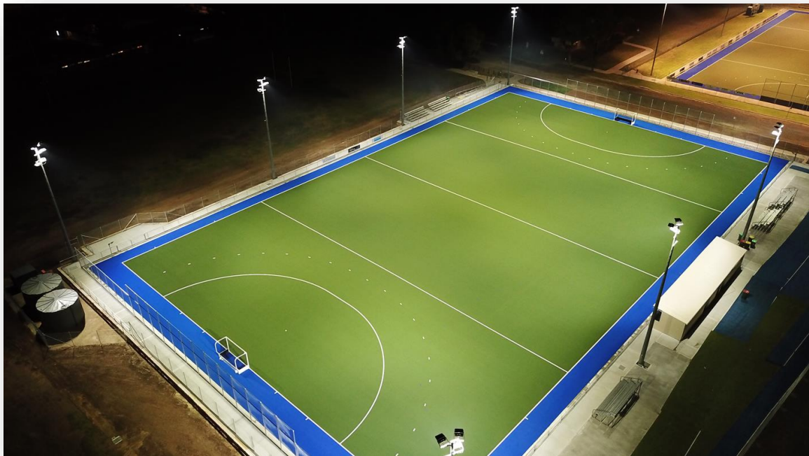
Photo 11 Testing of new LED lighting at the completed Stephen Davies Field.
