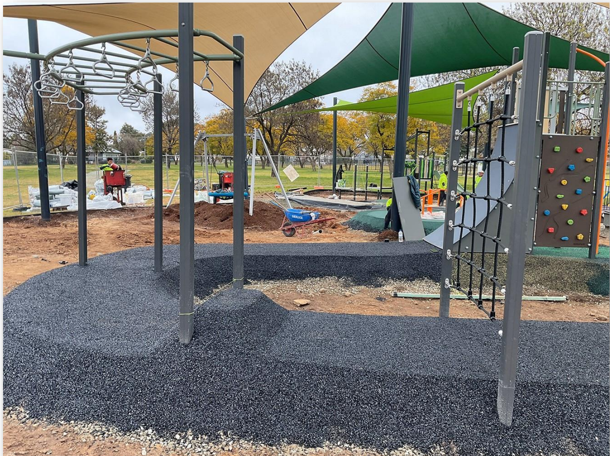
Photo 13: Kelly Reserve Ninja Park Under Construction
