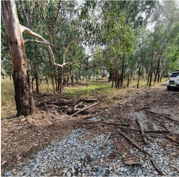
Plate 1 Existing crossing on access road
