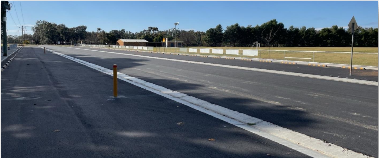
Photo 4 Drainage, carparking and footpath works at Harrison Park
