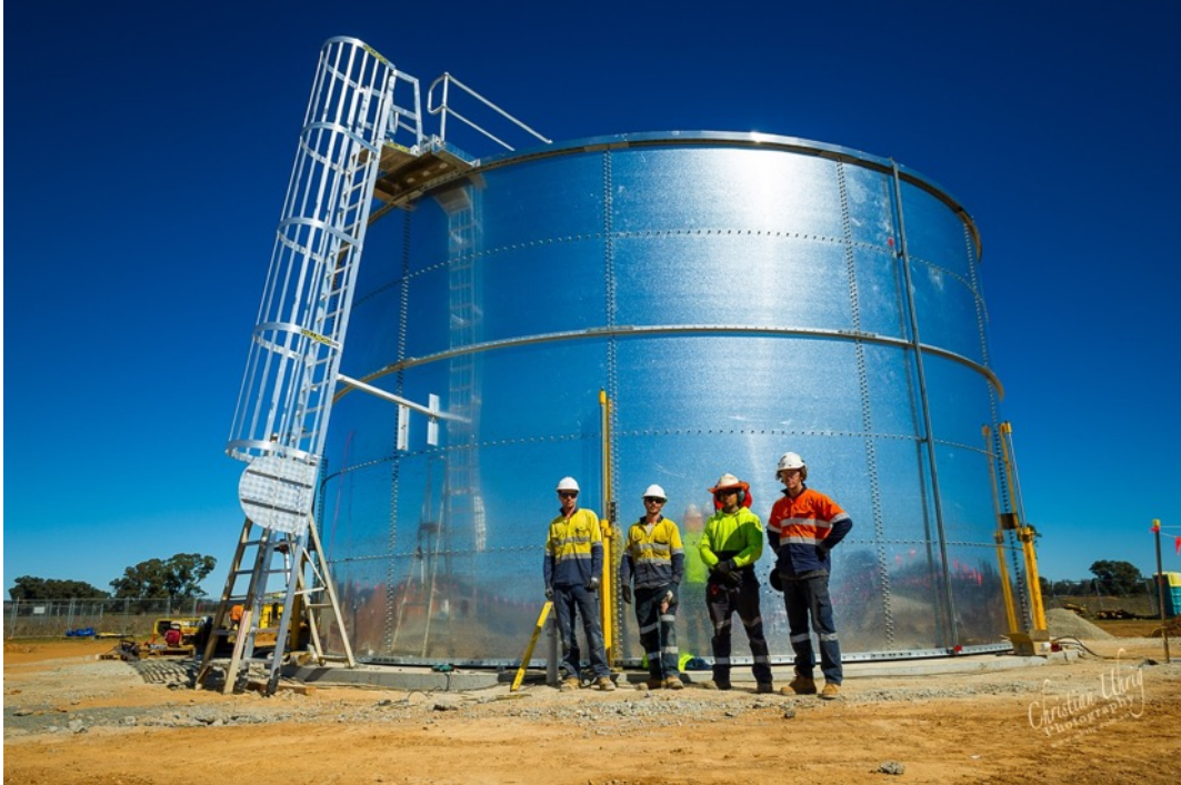
Advanced Water Recycling Facility under construction
