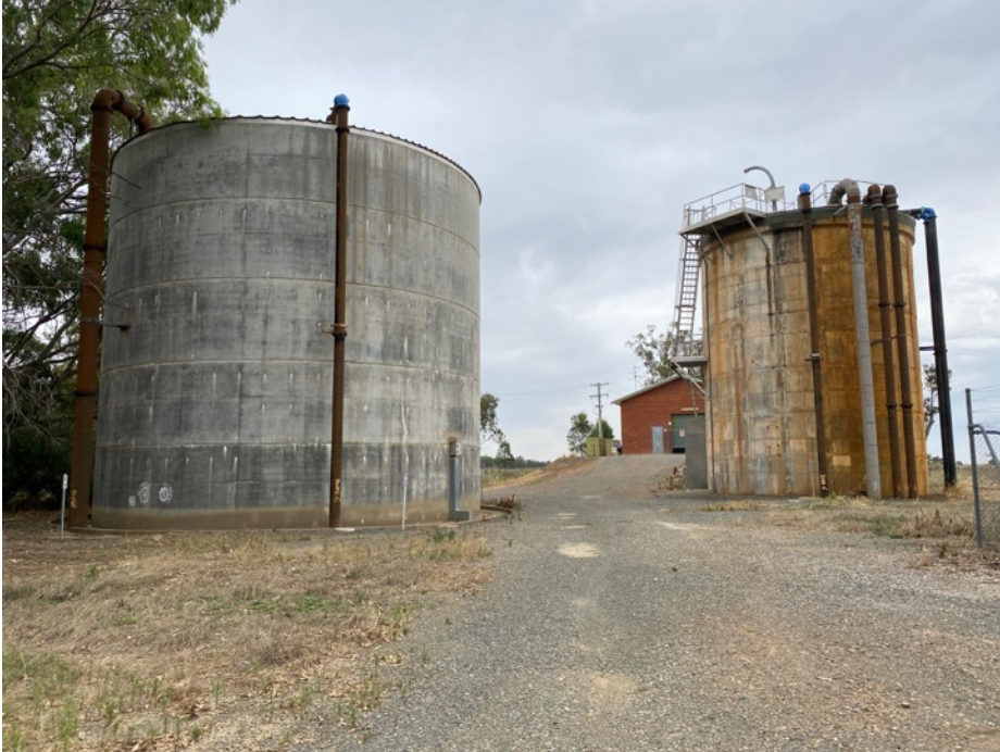
Figure 4-22: Eugowra Road Reservoirs
