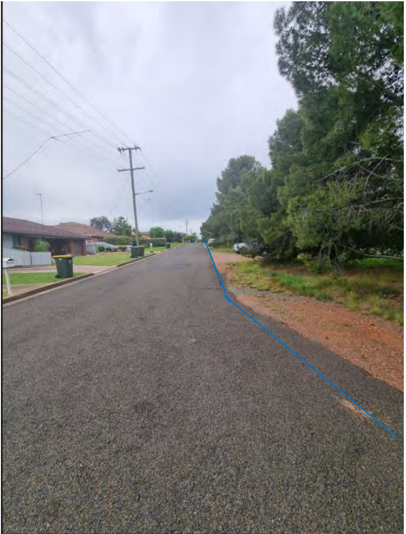
Figure 5.6 Clarinda/Henry Parkes Way crossing – Russell Street looking north
