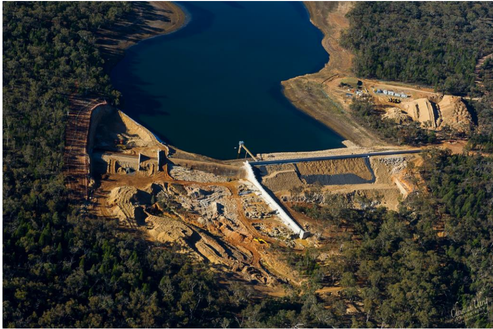
Lake Endeavour Dam Safety Upgrade – July 2014
