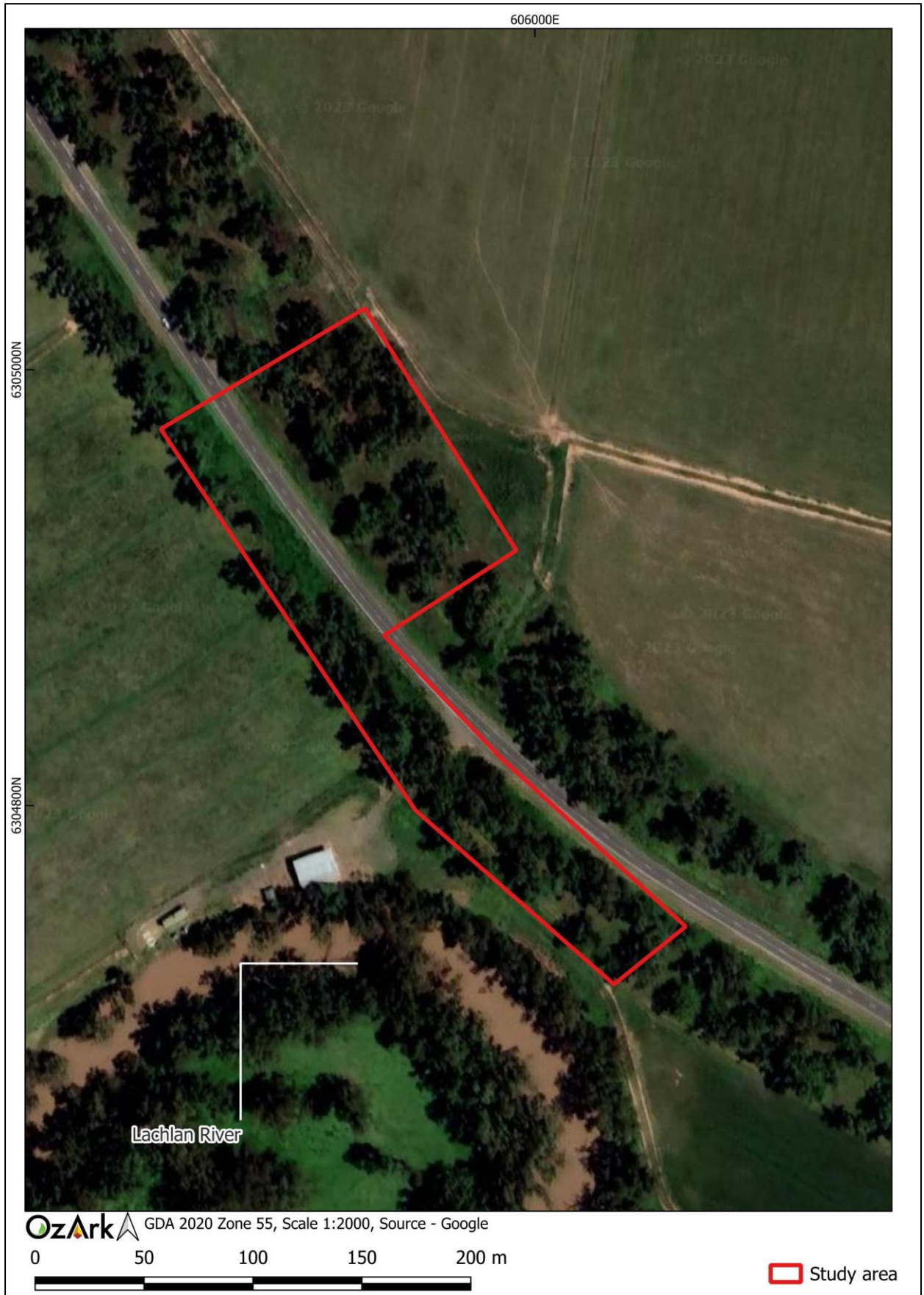
Figure 1-2: Aerial showing the study area.
