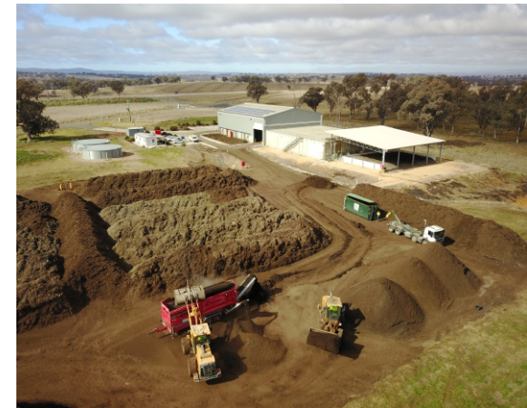
Euchareena Road Resource Recovery Centre
