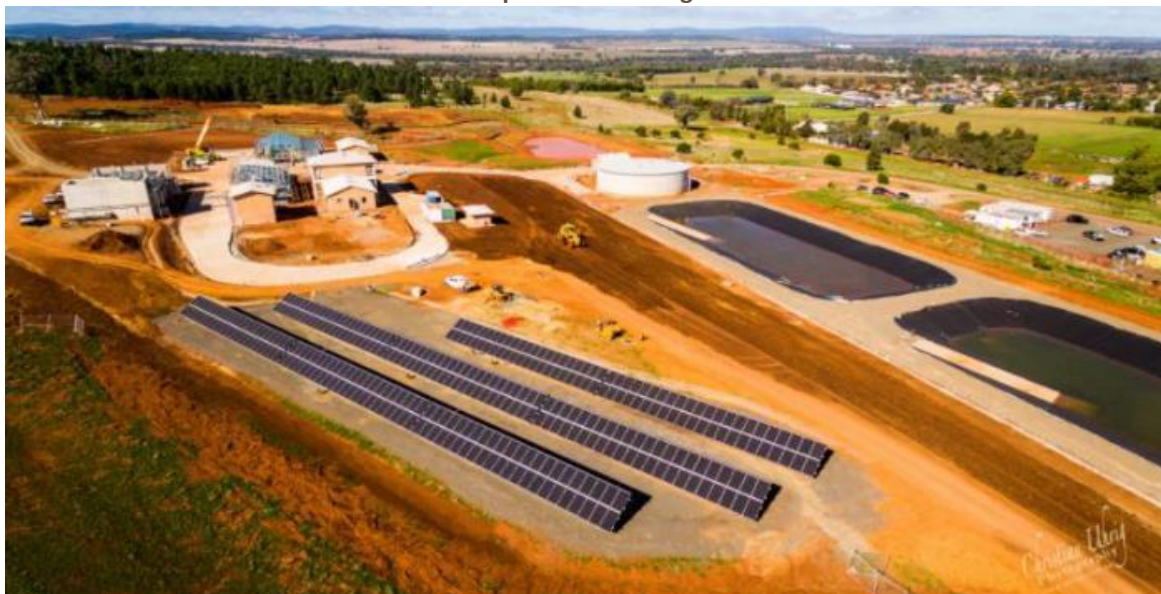
Plate 8 Aerial view of existing WTP (photo credit C Uhrig)
